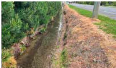
An intermittent roadside drain with gravel substrate embedded within fine sediment. Intermittent waterways are typically dry during summer months but flow more consistently during autumn and winter.
