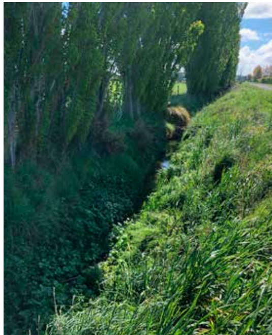
Where roads are elevated above the adjacent land, there may be very steep banks and little space within the road reserve for bank reshaping.
