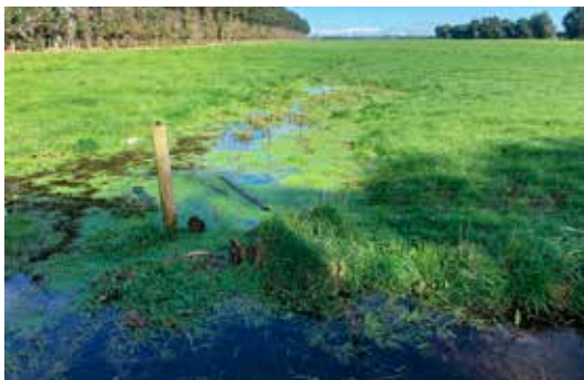
Springs that are unfenced can become pugged and become a source of sediment.
