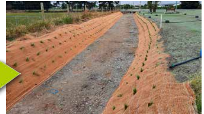
An example of a two stage channel – the Leeston Stormwater Bypass. Image source: SDC
