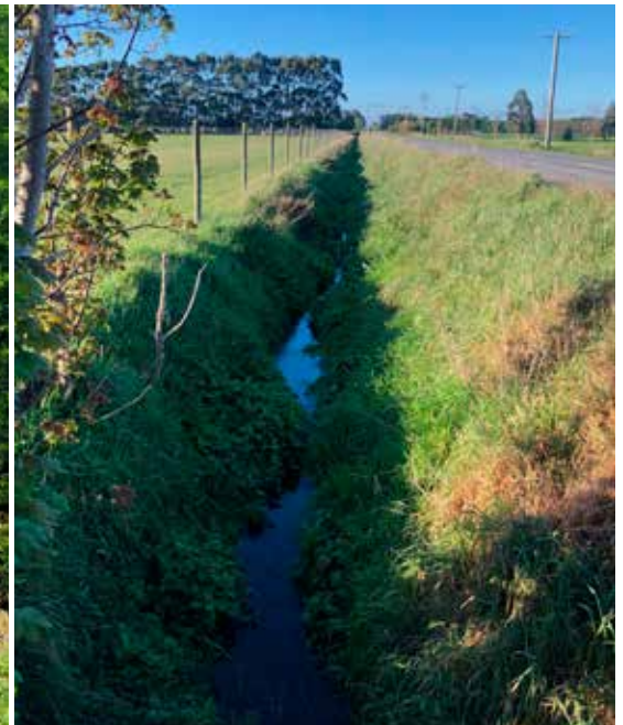
Roads and fences sited close to the drainage channel leave limited space for reshaping and planting.
