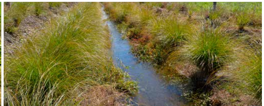
A recently planted two-stage channel showing the characteristic lower flood plain and steeper slopes of the upper banks (top), with the same channel shown below with the Carex secta becoming established and providing greater cover at the margins of the waterway.
