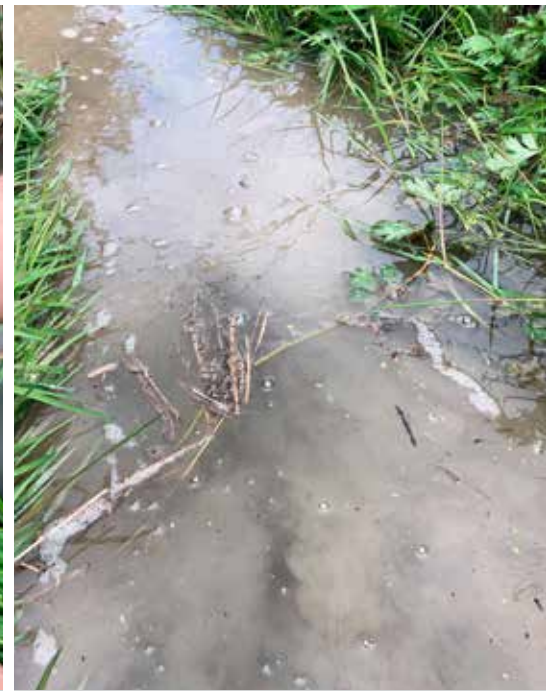
Suspended sediment in a drainage channel, stirred up from sediment within the channel itself.
