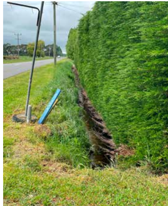
Powerlines are often located within 1 to 2 m of the top of existing banks, making bank reshaping a challenge.
