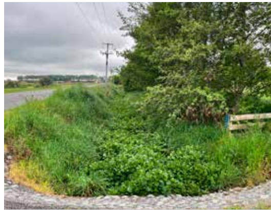
These drain channels are also obscured with emergent macrophytes.
