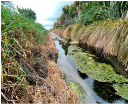
Steep banks that are slumping and inputting sediment to the waterway/drainage channel.
