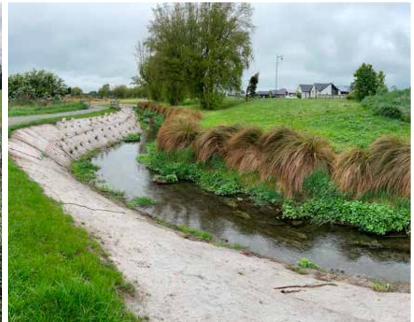
The close placement of cycleways/walkways within urban areas means that bank reshaping for bank stability is not always possible.
