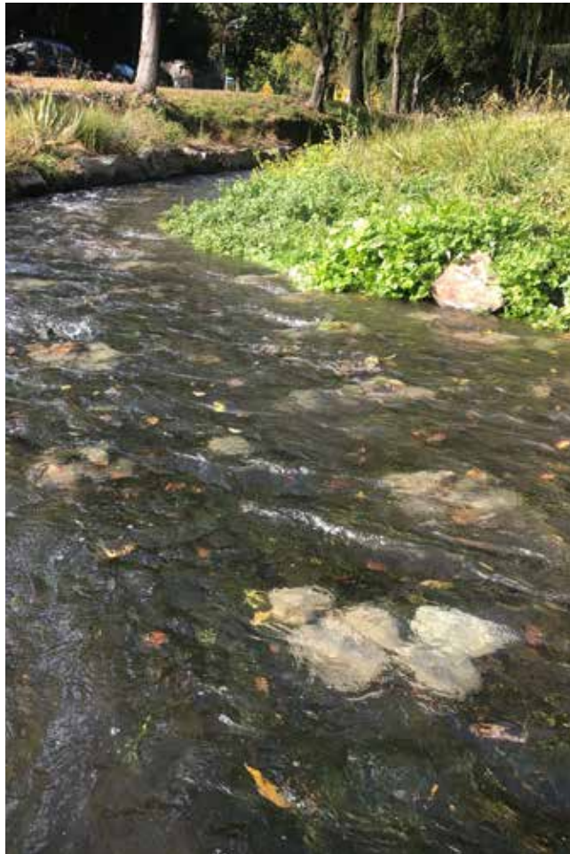
An array of cobble clusters increases instream habitat diversity for invertebrates and fish in gravel bed waterways.
