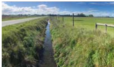
Steep banks and a lack of space for bank reshaping are known issues for intermittent drains.
