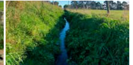
Perennial drains may have steep banks and little space for bank reshaping.
