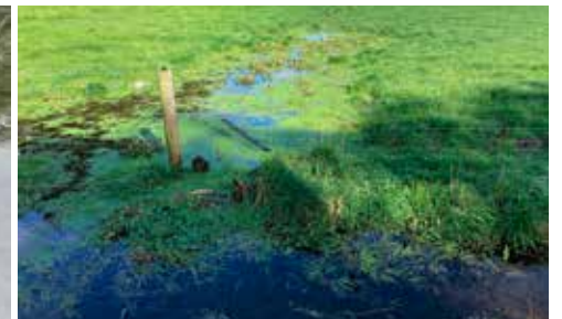
A springhead discharging to a nearby drainage channel.
