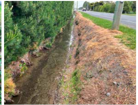
Banks that are regularly sprayed are an ongoing source of sediment to the drainage channel.
